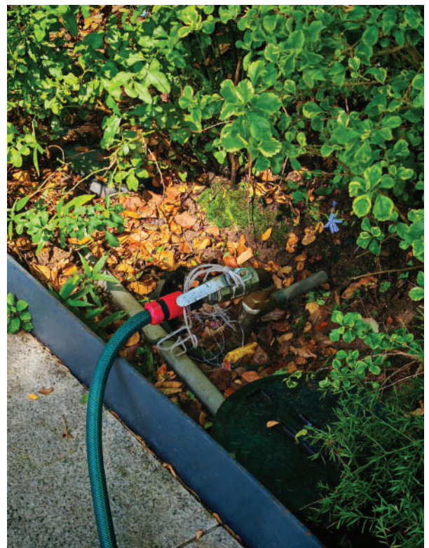
Rainwater outlet which dispenses collected rainwater for landscape irrigation
