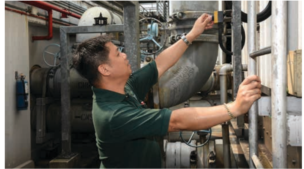
Regular monitoring and analysis of our utilities consumption allows Esplanade to achieve operational efficiencies.
